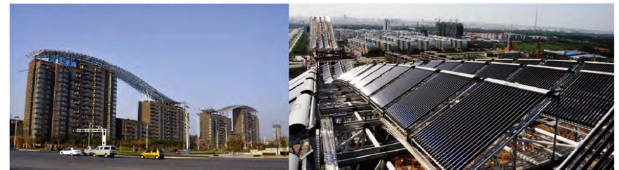
Himin's solar heating & cooling project for high-end residence property
