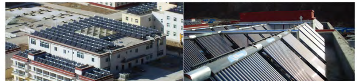
Himin's solar heating program for the first Tibetan hydropower plant
